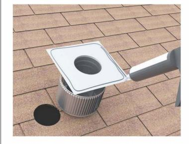
saw cut out a hole in the roof deck and remove all debris.
