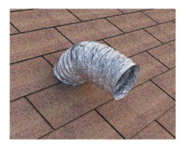
Step 7: Using a Zip Tie secure the Flex Duct to the Tail Pipe.
