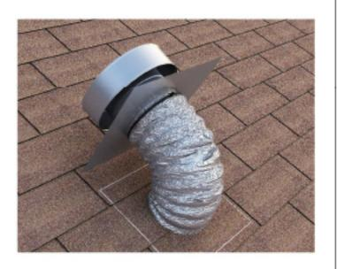
Step 8: Put roofing sealant on the underside along the bottom edge of falnge as shown
